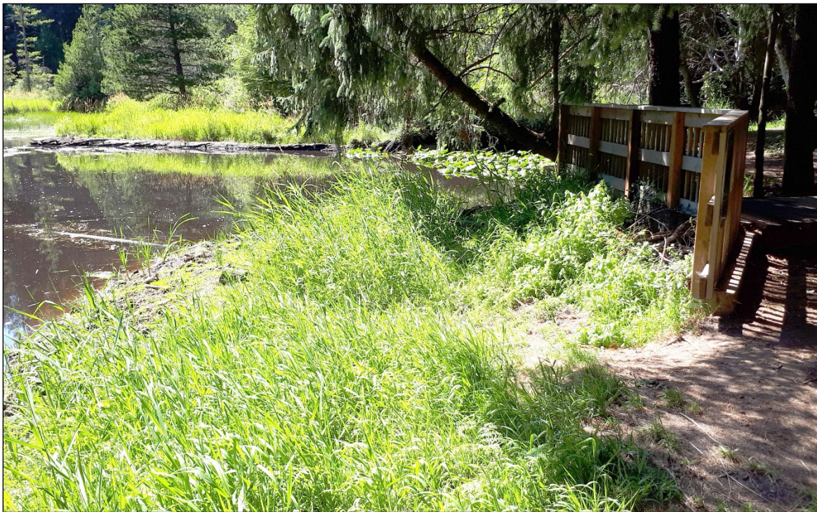
Figure 14: Capes Creek dam
